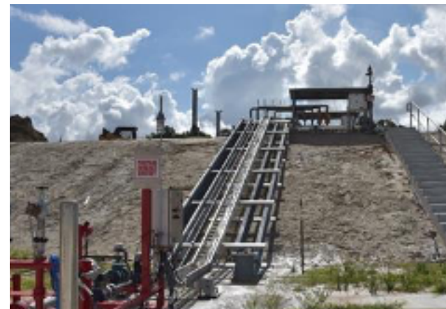
Bluebonnet Point Reserve will provide propane and air mixed with natural gas during peak demand periods.
