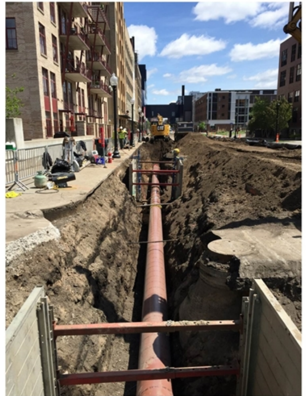
2015 Minnesota Beltline Replacement Project in downtown Minneapolis
