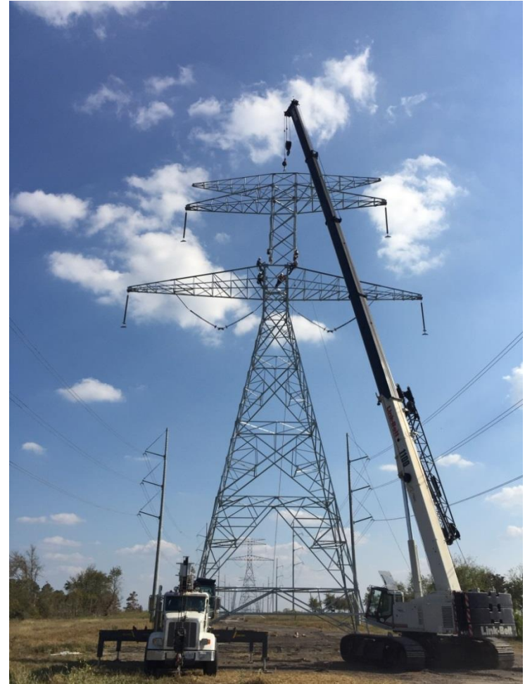
Construction of a new 345kV double circuit tower
