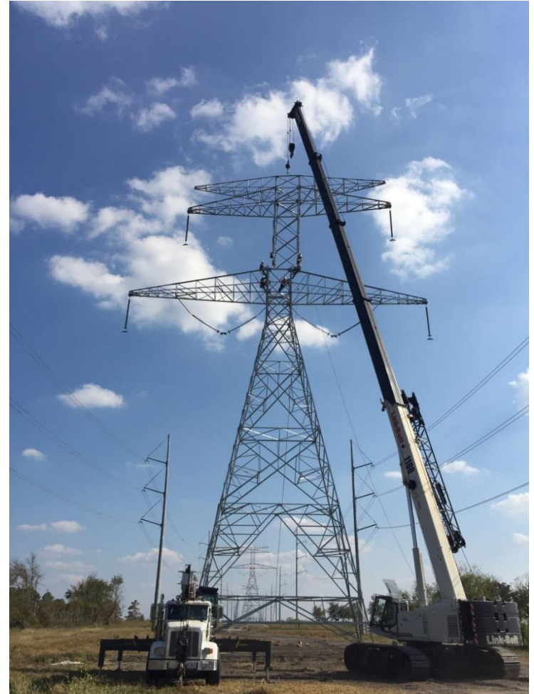
Construction of a new permanent 345kV double circuit tower in between temporary bypasses constructed to safely reenergize circuits damaged by tornadoes in April 2015.
