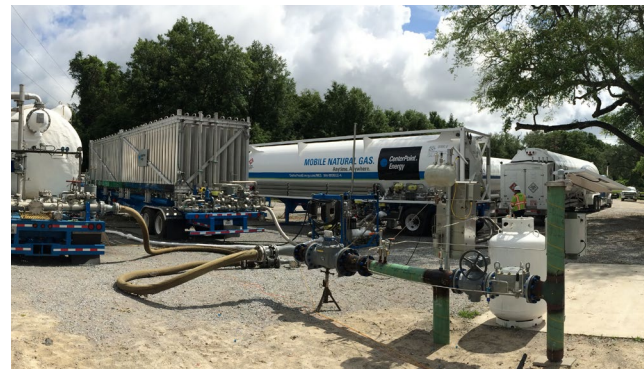
CenterPoint Energy Mobile Energy Solutions safely and reliably delivers mobile compressed natural gas and liquefied natural gas, eliminating interruptions caused by planned pipeline maintenance, construction or emergencies.
