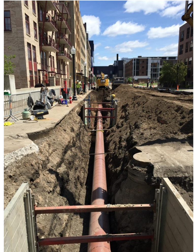
2015 Minnesota Beltline Replacement Project in downtown Minneapolis
