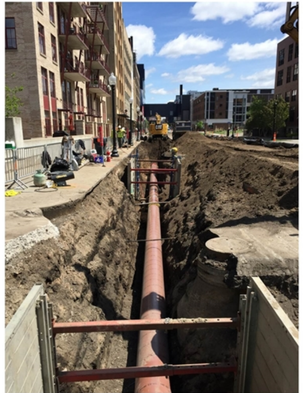
2015 Minnesota Beltline Replacement Project in downtown Minneapolis
