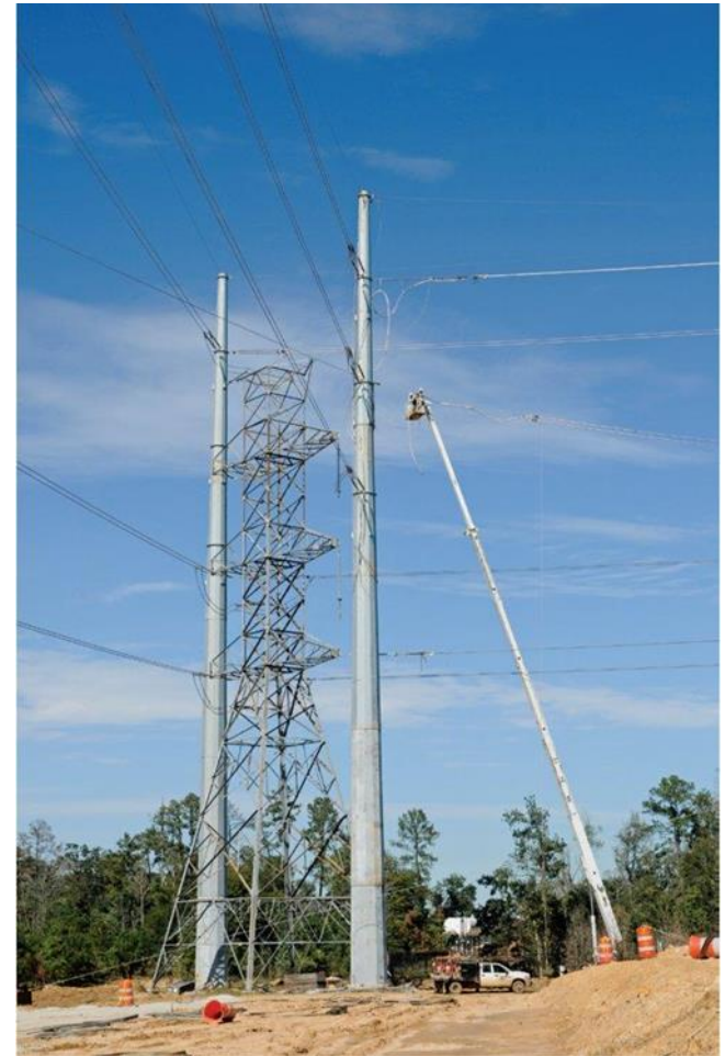
Construction of high voltage transmission infrastructure
