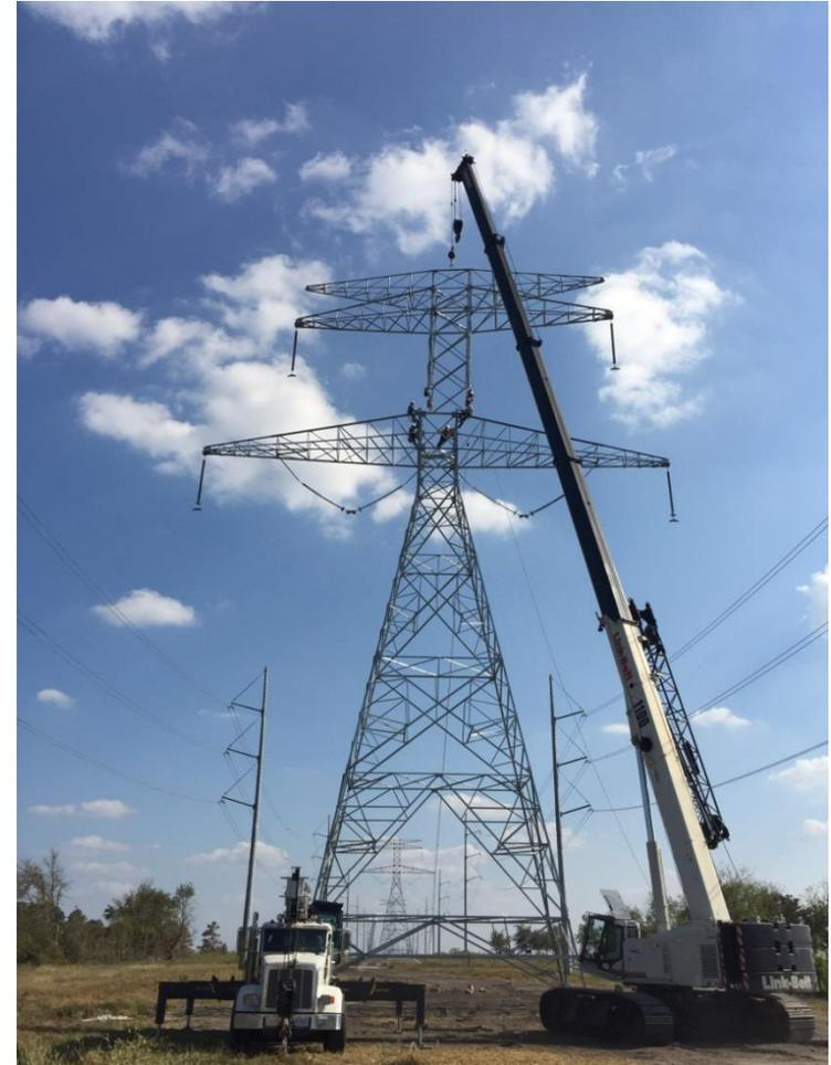
Construction of a new permanent 345kV double circuit tower in between temporary bypasses to safely reenergize circuits damaged by tornadoes in April 2015.
